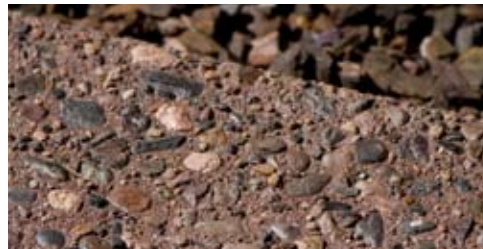
For the courtyard areas, Top-Cast™ 250 grade was applied to create a consistently high-quality deep exposed textured appearance.
