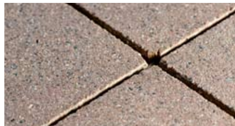
Top-Cast™ 03 etch-grade top-surface retarder was used to create an "acid-wash" like finish on CityNorth's sidewalks – without the traditionally cumbersome acid-wash process.
