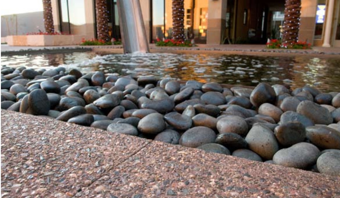
For the courtyard areas, Top-Cast™ 250 grade was applied to create a consistently high-quality deep exposed textured appearance.
